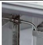
Water is filled in a drip box behind the air conveyor grid.
